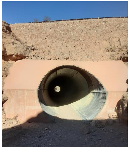
EXAMPLE OF A CORRUGATED METAL TRAIL UNDERPASS
